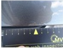
Foglight L, Crack, E - Replace
