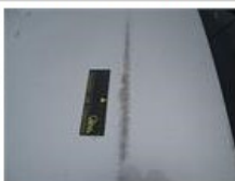
Roof, Scratch(es), LI - Repair and paint (complete)
