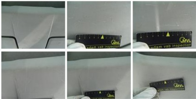
Bumper F, Broken, E - Replace 398,40
