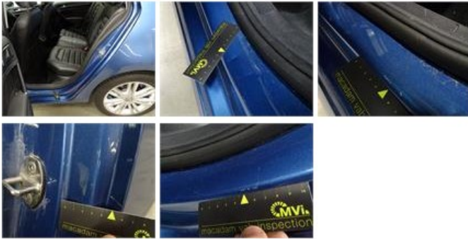
Sill outer L, Dent(s), LI - Repair and paint (complete)
