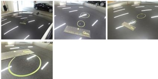
Protection plate M, Tear, E - Replace
