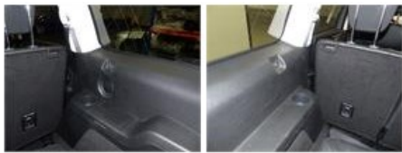
Spoiler R, Deformed / Strained, E - Replace
