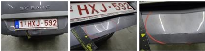
Bonnet, Bad repair, Acceptable
