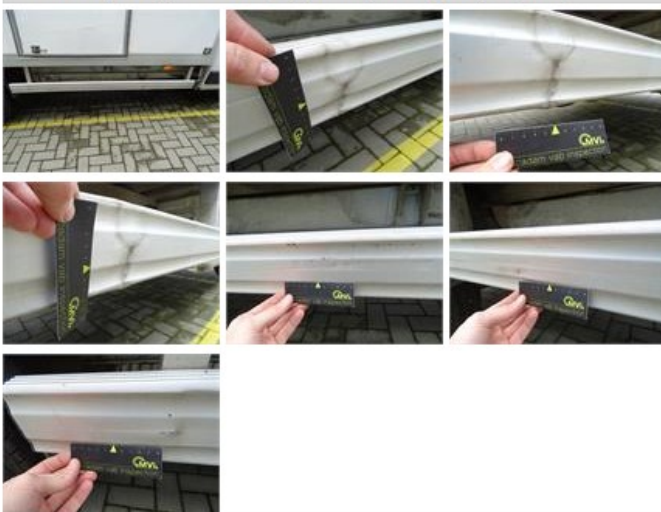
Sill trim F R, Broken, E - Replace
