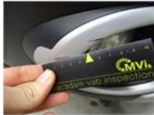
Roof, Dent(s), Acceptable
