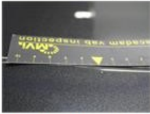
Door F L, Bad repair, Acceptable
