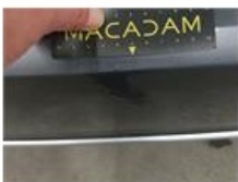
Interior, Not original part, Acceptable
