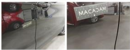
Interior, No damage, Acceptable
