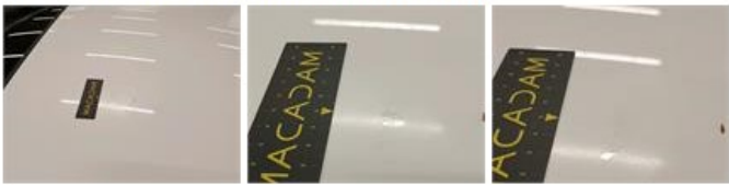
Door RR, Repaired, Acceptable
